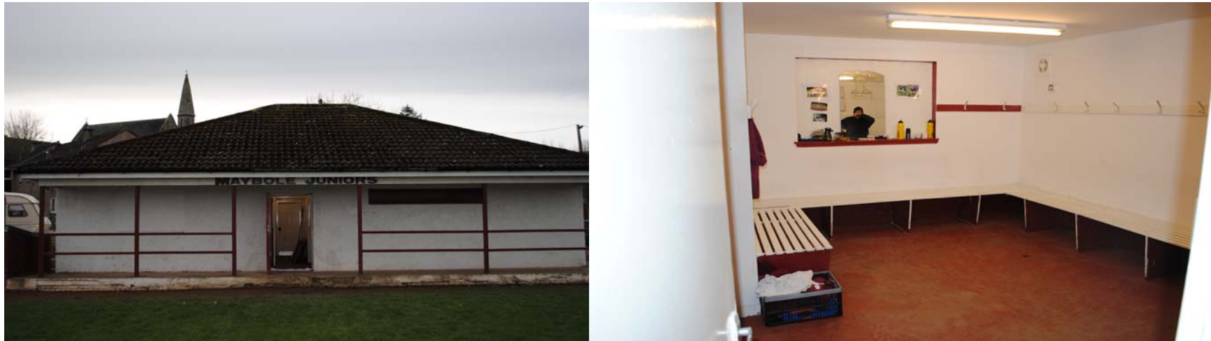
Maybole Juniors Changing Rooms and main office, above. Spectator Stands and playing field (showing evidence of sinking), and spectator toilets, below.
