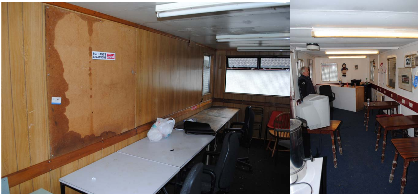
Portacabins following storm damage, above, and main hospitality room.
